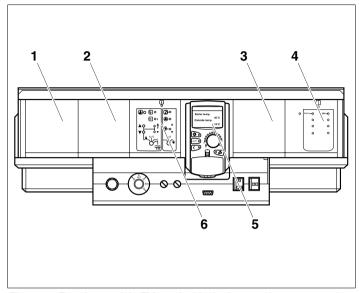
Function module FM 446 inside the Logamatic 4311 control Fig. 5 device
